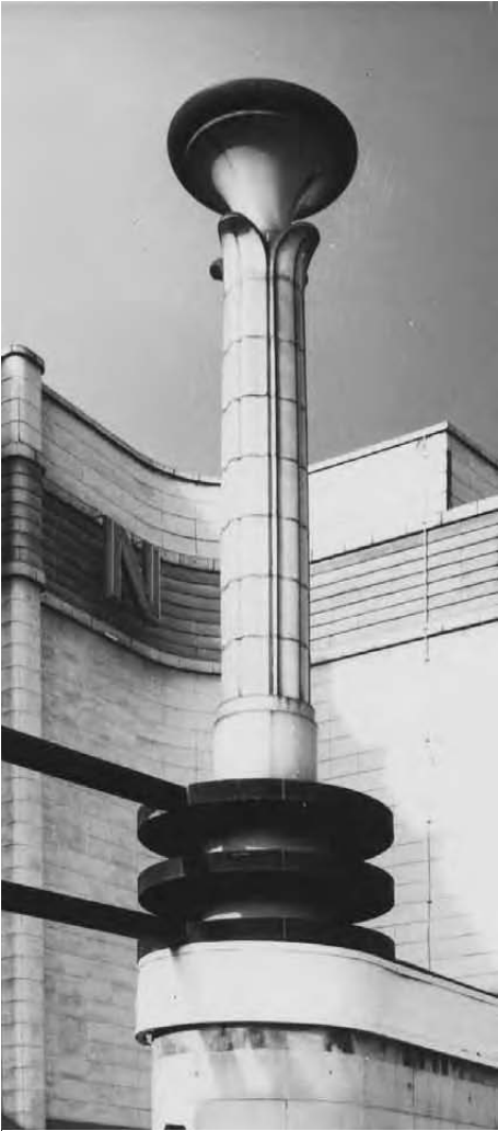
Plate 215 Detail of a lamp-standard from the Odeon Cinema at Woolwich, London, with Egyptianising ornament in faïence. Photograph of 1973 (GLPL No. 73/11290).
